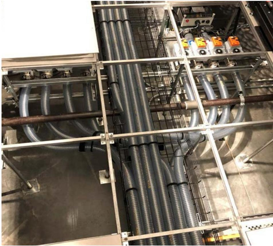
Figure 4: Chillydyne Installation at Sandia National Laboratory
